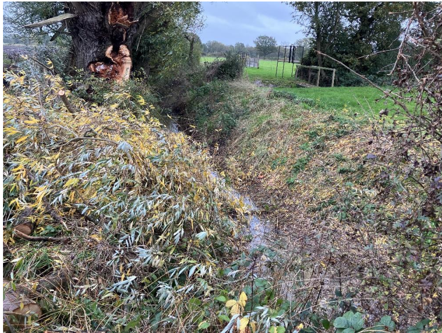
Plate 9-6: Ell Wood and Fenwick Grange Drain, looking downstream (8 November 2024)
